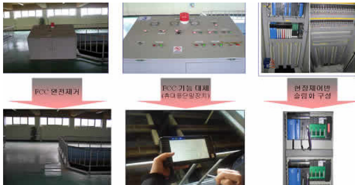
SLIMMER INDEED! Comparative photos, showing how (top rows) the older plant equipment and cabling have been replaced by PROFIBUS-based equivalents (bottom rows), saving space, time and cost.
